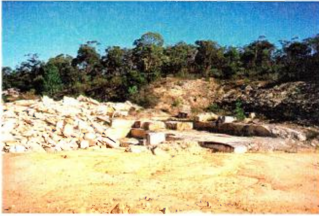
Filling with overburden
